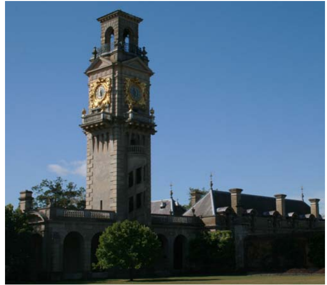
Figure 5. Cliveden, Buckinghamshire: ornate tower built in 1861 to hold water for fire hydrants and domestic use
