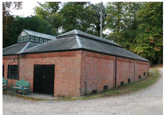
Figure 2. Ascott, Buckinghamshire: buildings erected in the 1890s for Leopold de Rothschild, housing a steam-powered electricity generating plant and sawmill. Nearby are the remains of private water works and sewage plant and an earlier gas works
