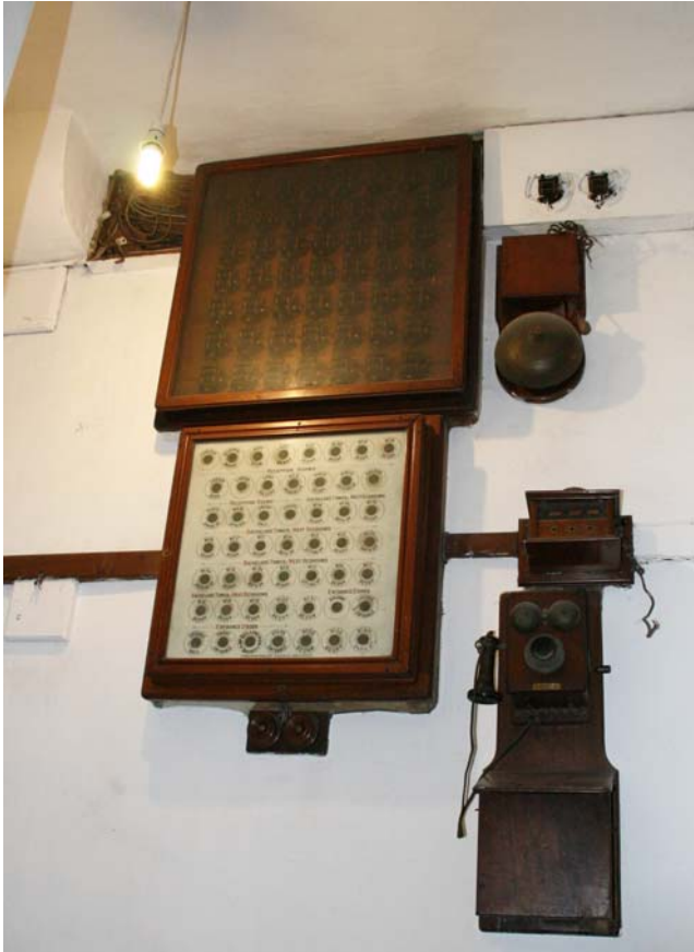
Figure 10. Chirk Castle, Clwyd: electric bell annunciator boards and internal telephone system
